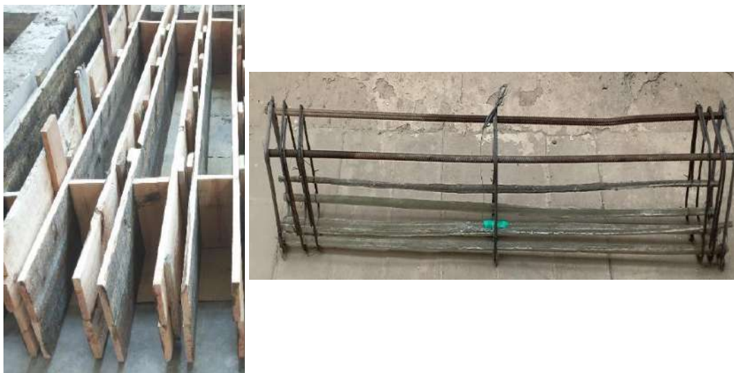
Fig. 4. Details of Reinforcement and Wooden Forms.
