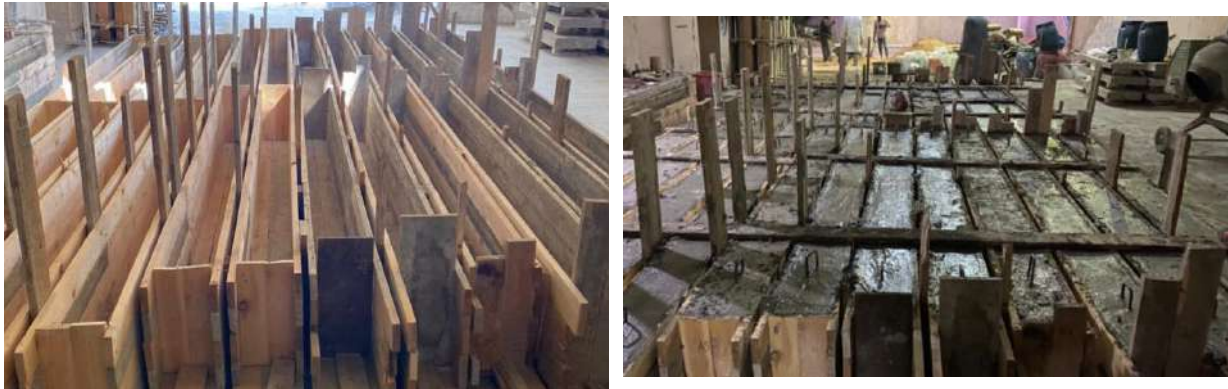
Figure 4. Fabrication process before and after casting
