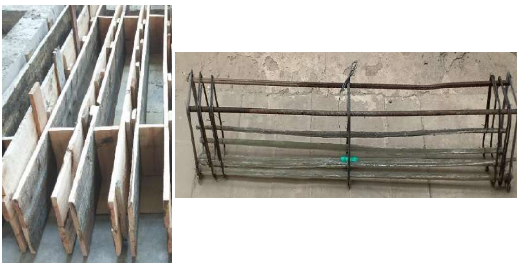
Fig. 4. Details of Reinforcement and Wooden Forms.
